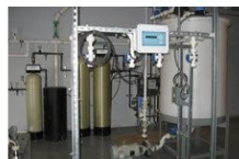
Underground workings - perfectly maintained and always operational
